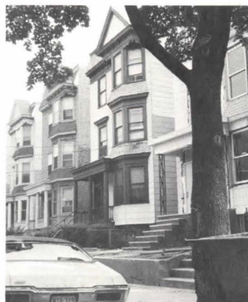
Typical rehab street
