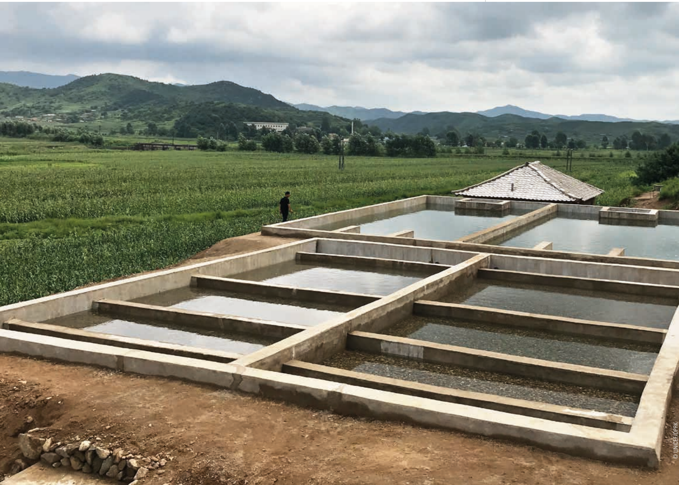
Water treatment system in DPR Korea
