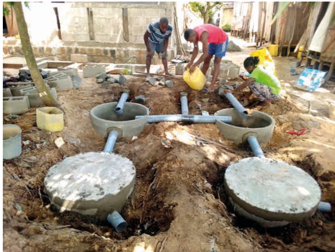
Latrine construction (with collection chambers) in Madagascar
