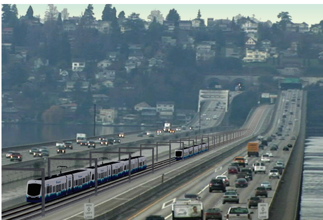
Simulation of Light Rail on I-90 with Completed I-90 Two-Way Transit and HOV Operations Project
