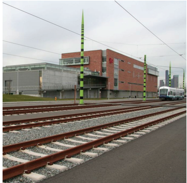
View of Sound Transit's Central Link Operations and Maintenance Facility in Seattle
