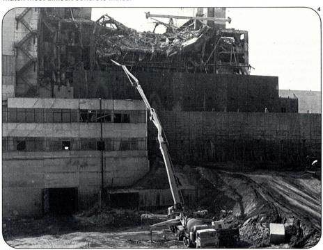
The 52 metre five section Putzmeister filling the middle step – steel form – of the pyramid entombment. This unit performed the outstanding 100,000 cubic yards within three months – the lion's share of the whole pumping job.
