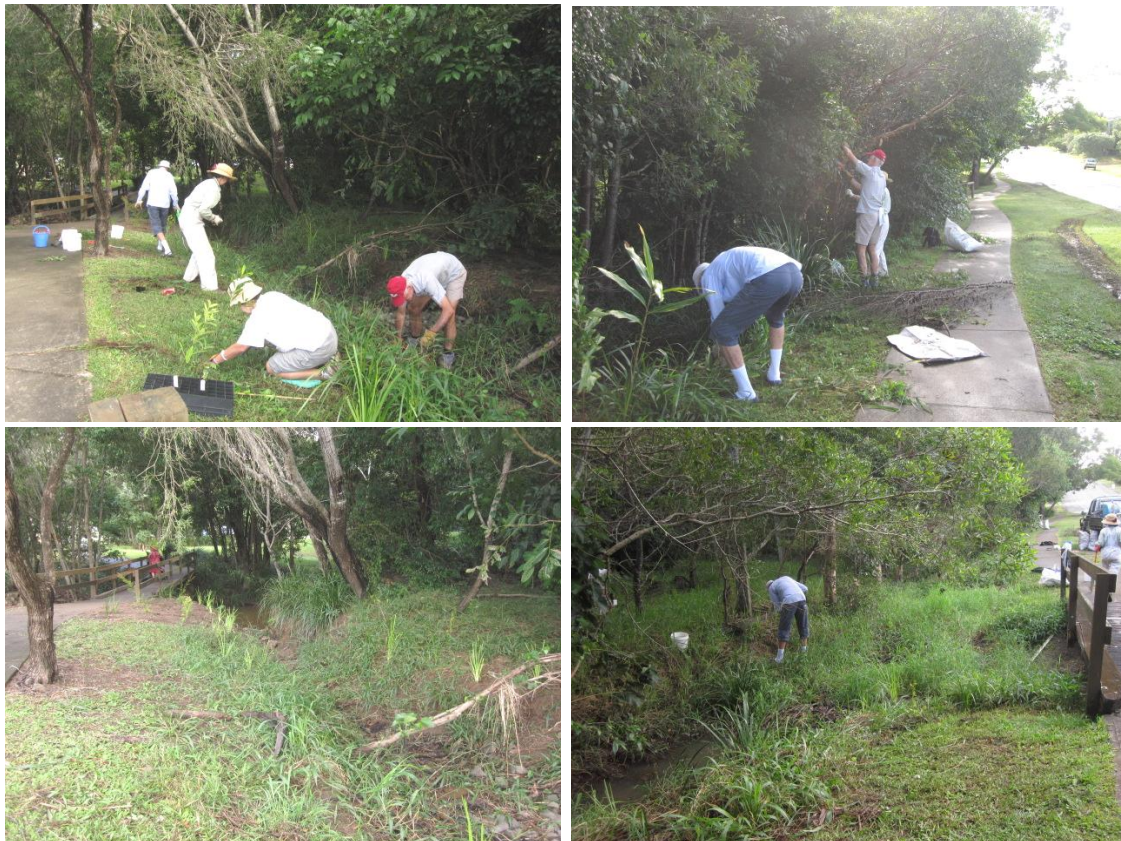
Photos 31-34 : Eighty plants were planted along the drain in Hill Street
