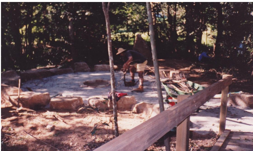
Photo 20: Construction of the Speaking Circle
