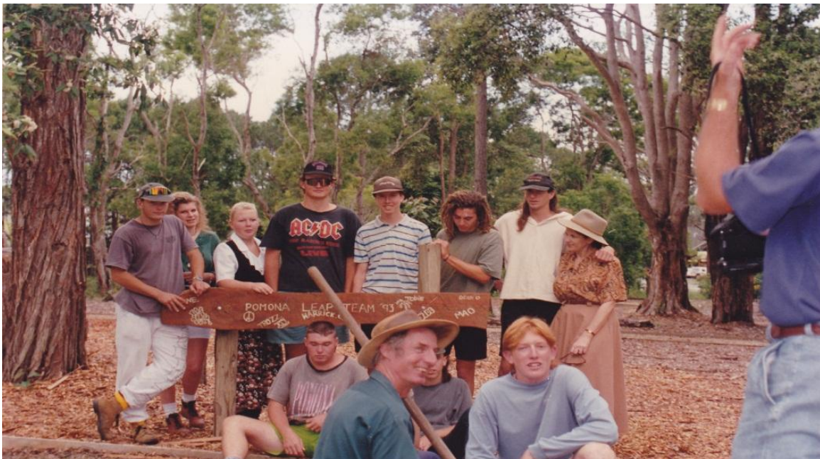
Photos 7 – 10: The LEAP Team involved in the construction of pathways in 1993
