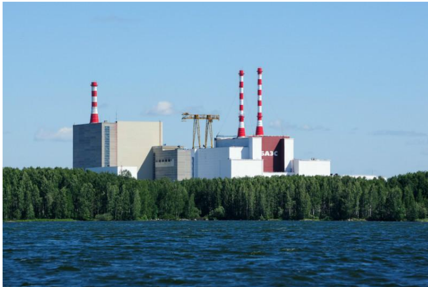
View from the water-storage reservoir to power units No. 1-3 of the Beloyarsk NPP
