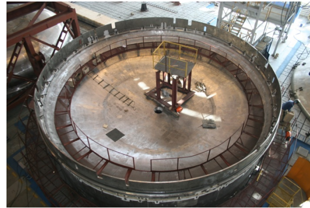
Mounting of the reactor vessel bottoms
