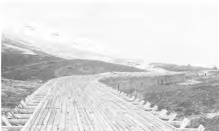
Snow tunnel on Reichsstrasse 50.
