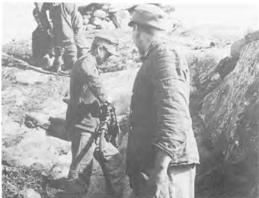
Engineer using jackhammer to break up rocks for the construction of positions on the Litsa River front.
