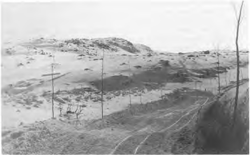
Snow-covered road in northern Finland. Note dead saplings placed to indicate outline of road.
