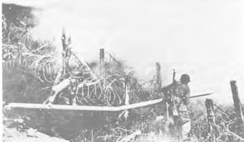
Finnish engineers using bangalore torpedo to demolish Russian fortifications on the Isthmus of Karelia.
