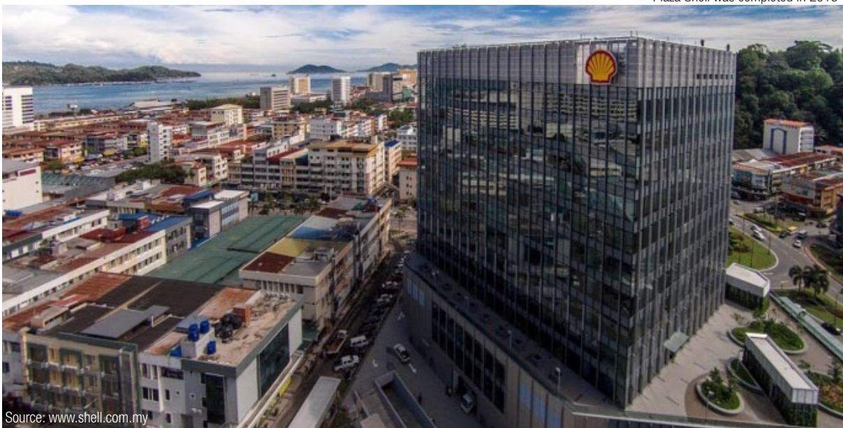
Plaza Shell was completed in 2015
