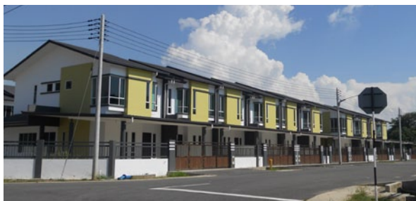
Double-storey Terraced Houses in Gem Park, Bintulu
