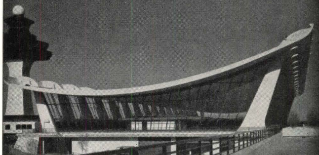
Dulles International Airport, Chantilly, Va. • Eero Saarinen Associates, Architects • Gacoflex Elastomeric Roofing System
