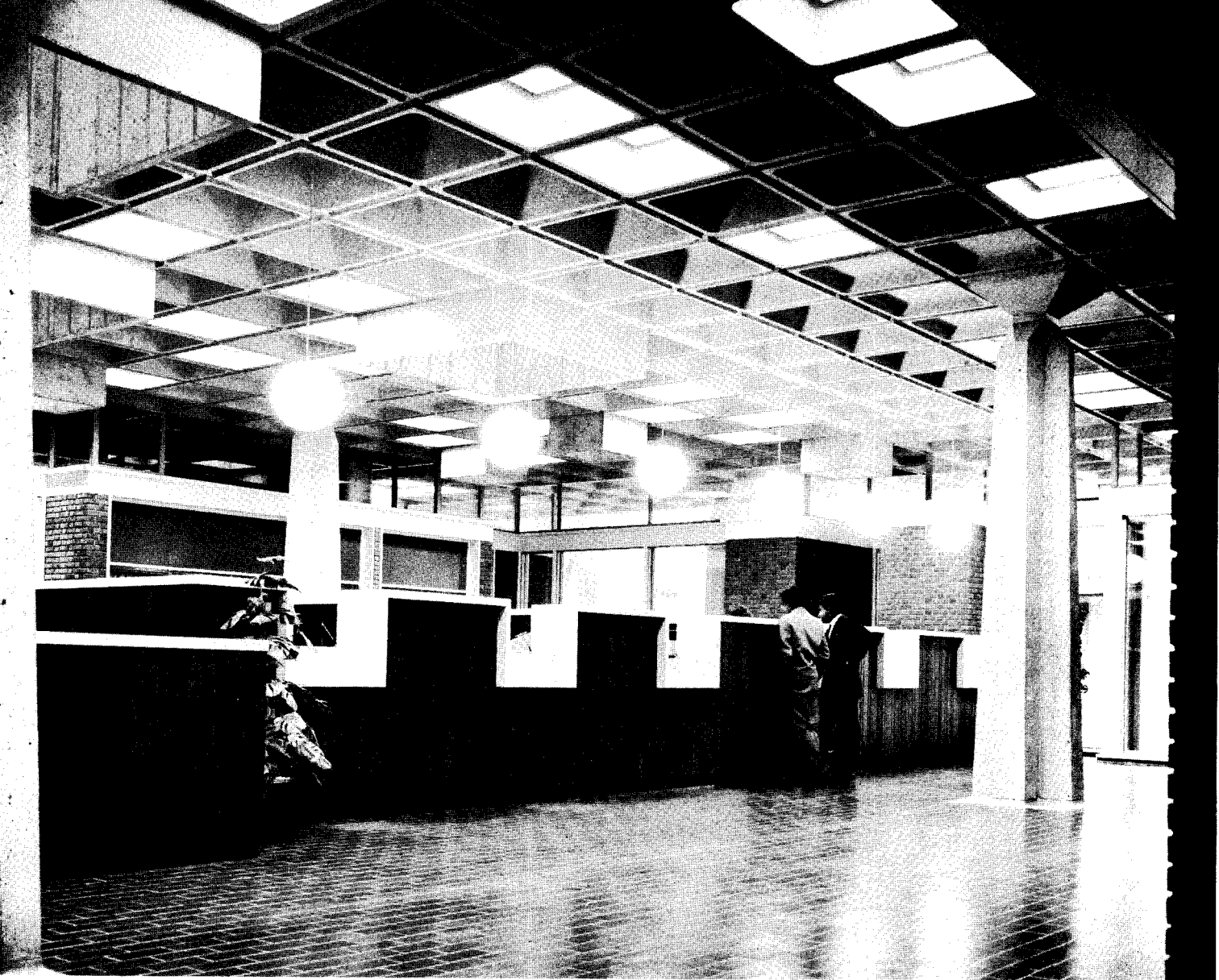
The wood front of the tellers' counter (above) repeats the random pattern of formwork used on the roof parapet and the podium (below). The floors are quarry tile; doors are oak-stained almost black. The meeting room on the basement level (left) has dark-stained vertical oak boards on the walls. The ceiling track across the center of the room is for a folding door. Molded cylindrical ceiling forms contain air-conditioning supply and lighting.
