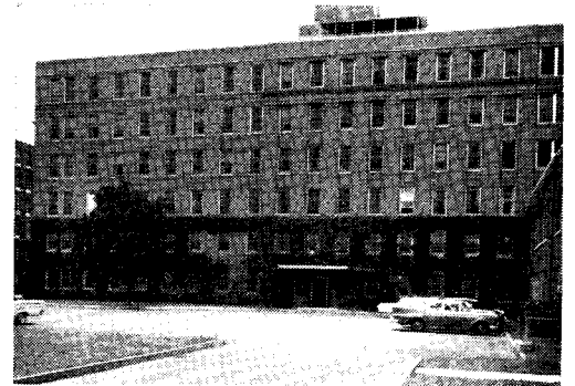
This hospital wing in Rochester, N. Y., was constructed in 1940.
