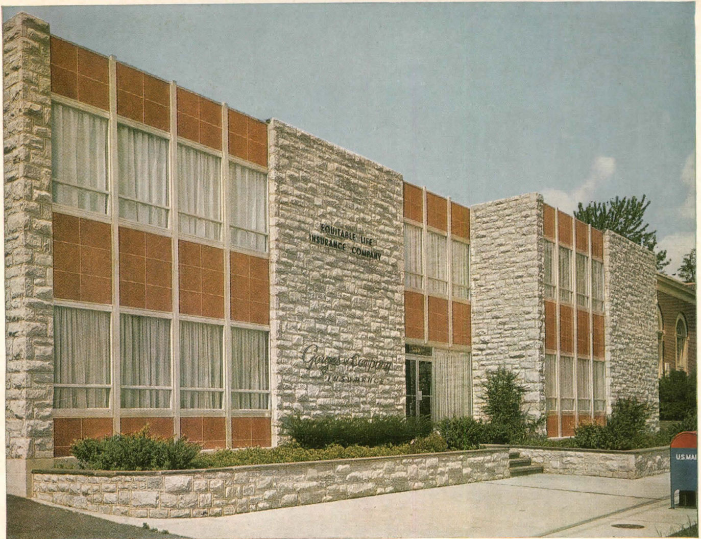
Office Building, Baltimore, Md. Thomas R. Silcox, architect. Lawrence Construction Co., builder. CV Durathin Insulated Panels in mottled cinnamon were specified in several sizes up to 4'6" x 4'. All panels are 1 7/8" thick with Foamglas insulation.
