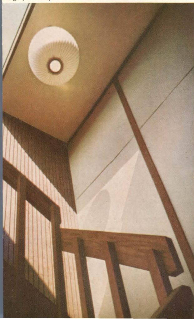
Large panels speed erection, lower construction costs.
