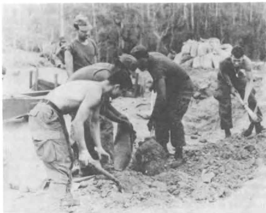
MEN FROM BATTERY A, 2D BATTALION, 319TH FIELD ARTILLERY, BUILDING PARAPETS
