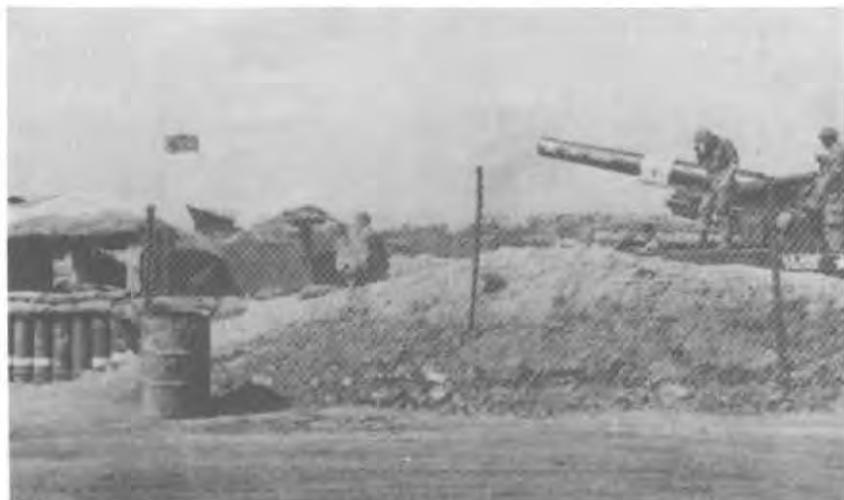
BATTERY D, 3D BATTALION, 13TH FIELD ARTILLERY, AT FIRE SUPPORT BASE STUART, JUNE 1969. Chain link fence has been installed for protection against B40 rockets.
