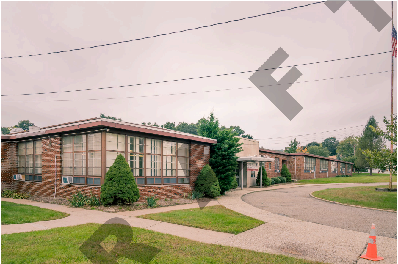
41. School: Facade, with lower wing (left) and entrance bay (right), camera facing northwest
