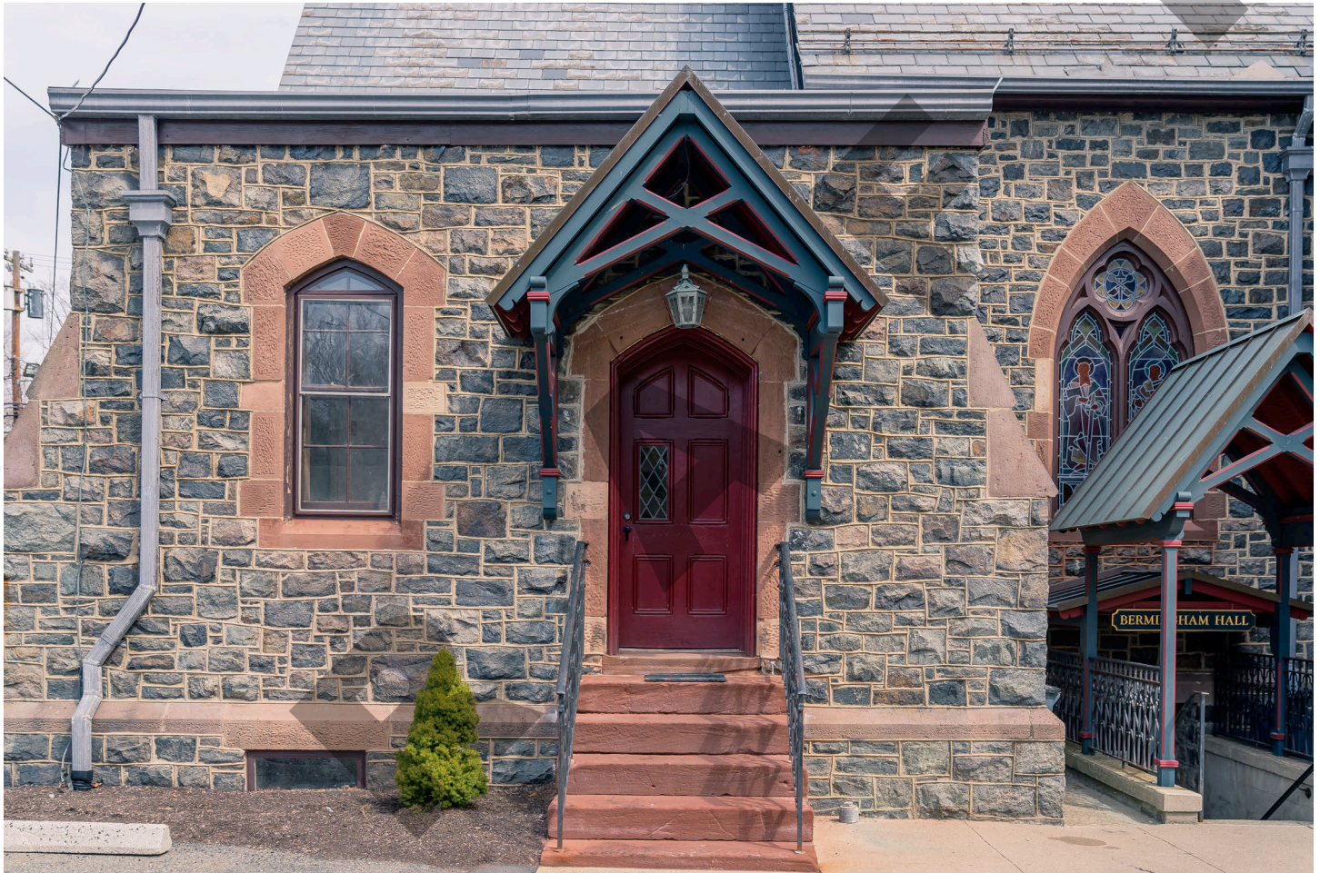
14. Sacristy and basement Hall entry, camera facing east
