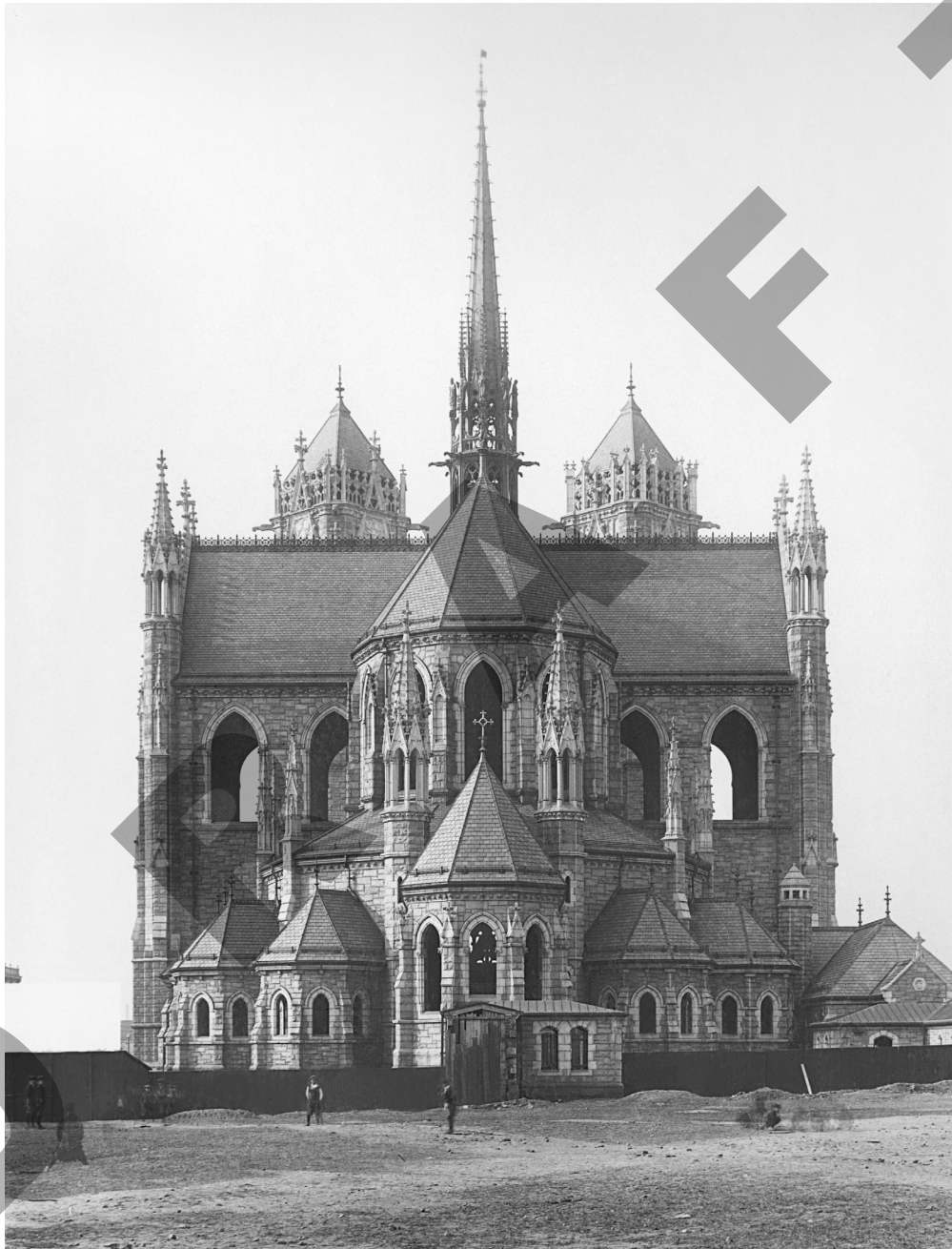
3. Jeremiah O'Rourke's Sacred Heart Cathedral, Newark, c.s. 1899, apse side under construction. Archives of the Archdiocese of Newark
