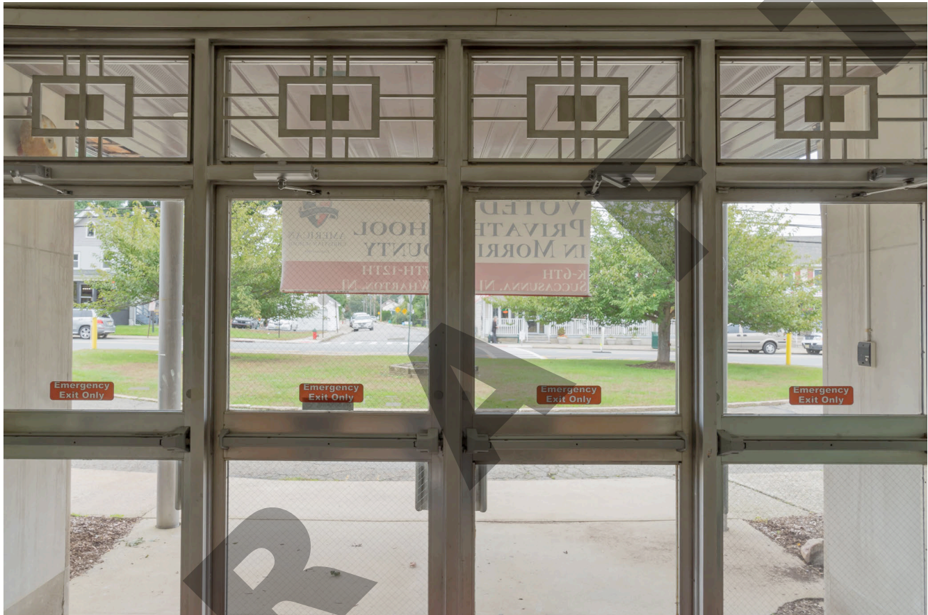
39. School: Entry from inside, with metallic grills, camera facing east
