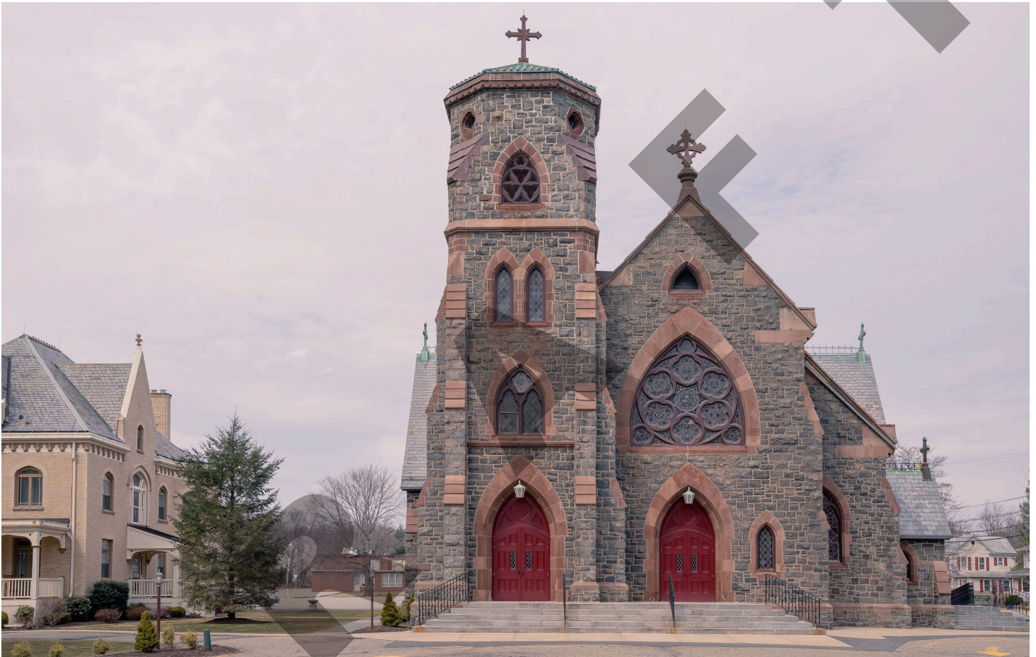
7. Facade, camera facing north
