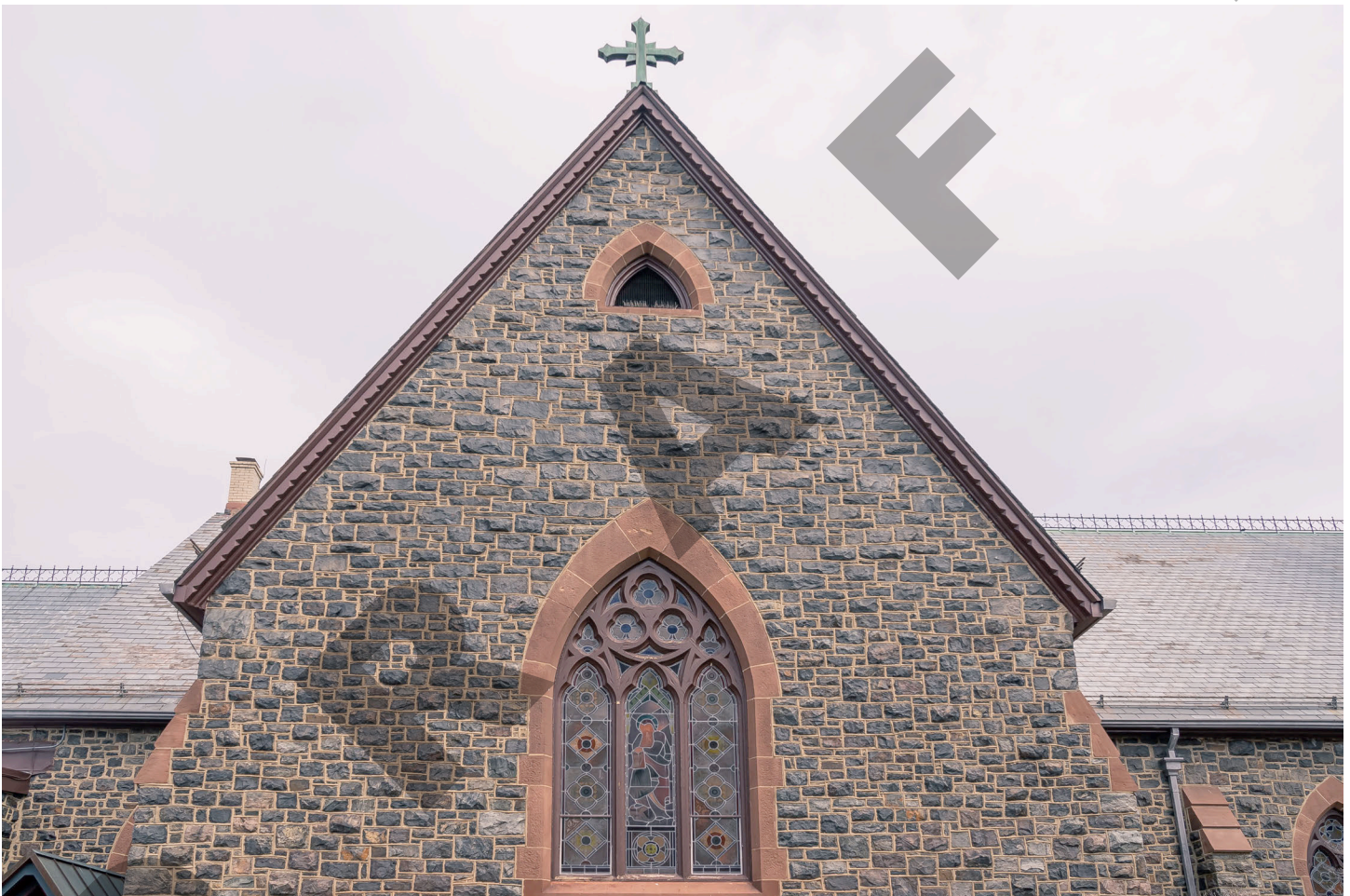
13. West transept wall showing stone work, camera facing east
