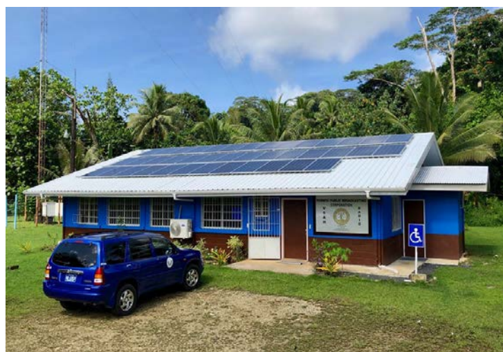
The 40 new solar panels on the V6AH radio station. Credit: IOM, 2019.
