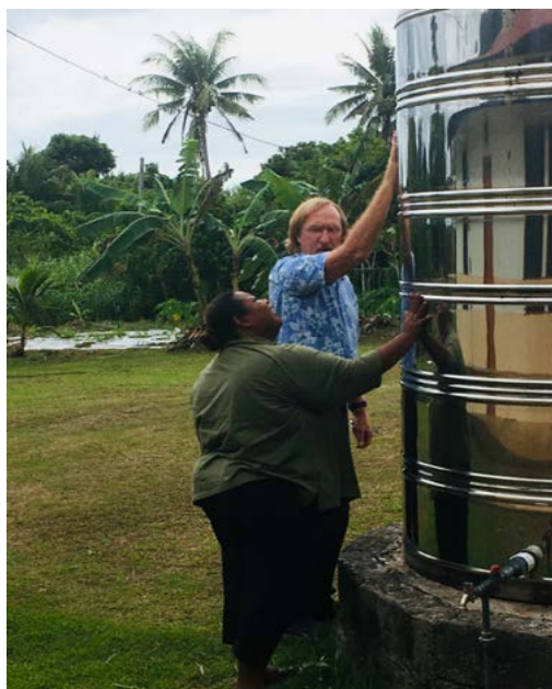
IOM staff Dale Jenkins shows a WQMT team leader how to check water levels by manually measuring temperature. Credit: IOM, 2019.
