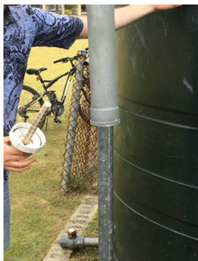
Alii CADRE staff member demonstrating the proper technique of cleaning the flush function. Credit: IOM, 2019.
