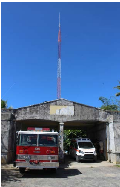
The re-erected antenna at the Pohnpei Disaster Coordination Building. Credit: IOM, 2018.
