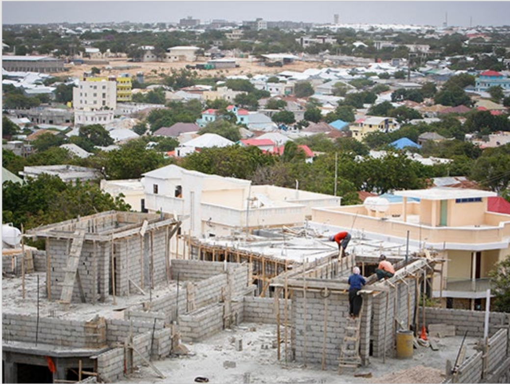
New building construction, Medina district, Mogadishu, Hirshabelle Flickr / AMISOM Public Information
