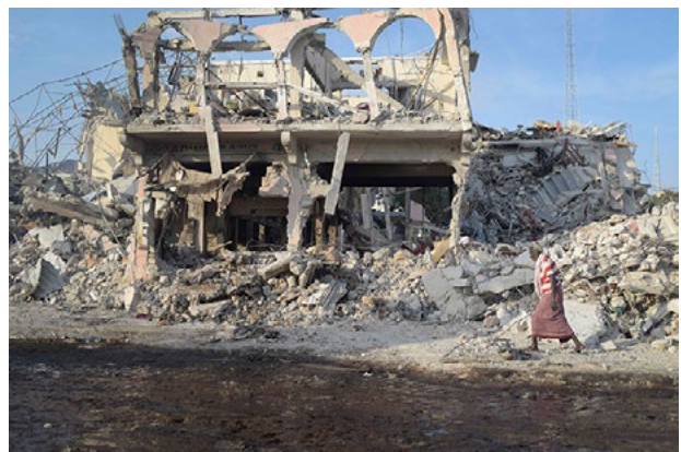
Collapsed building, Mogadishu, Hirshabelle Flickr / AMISON Public Information
