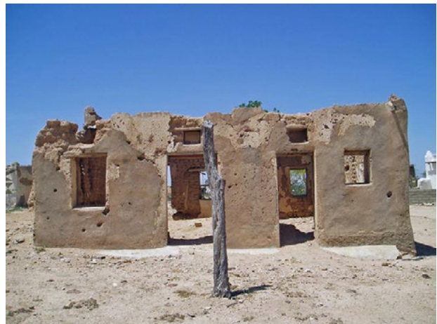
Remains of houses damaged by war, Hargeysa, Somaliland Flickr / najeeb
