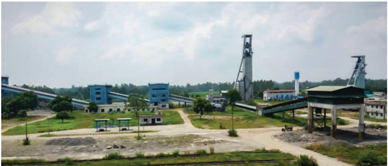
Cage Skip Shaft and Crushing Plant of MGMCL
