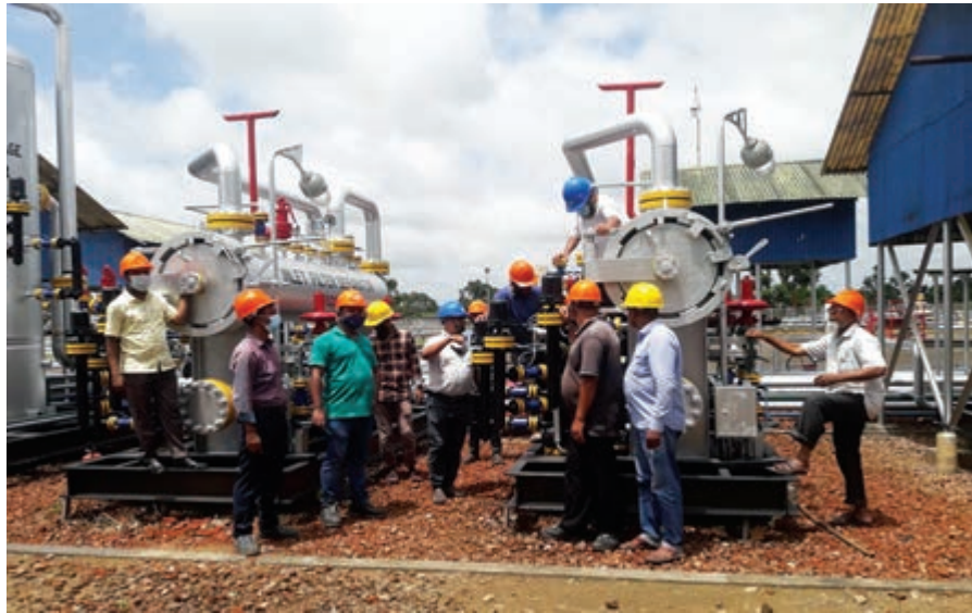
Maintenance work at Rashidpur Gas Field of SGFL
