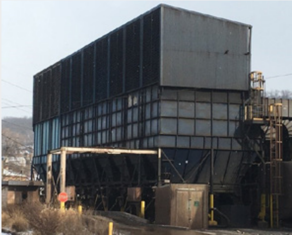
Figure 18. BOP fugitive baghouse.
