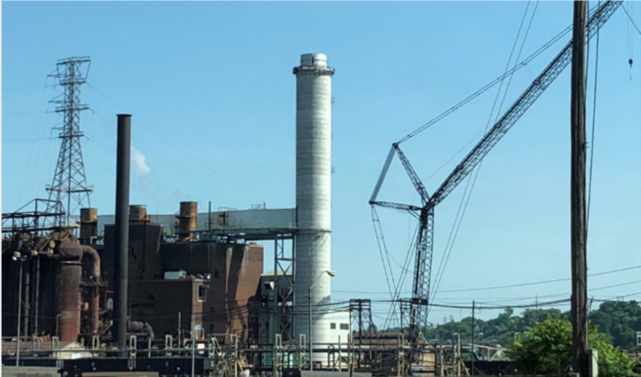
Figure 25. The newly constructed Edgar Thomson boiler stack was built to improve dispersion.
