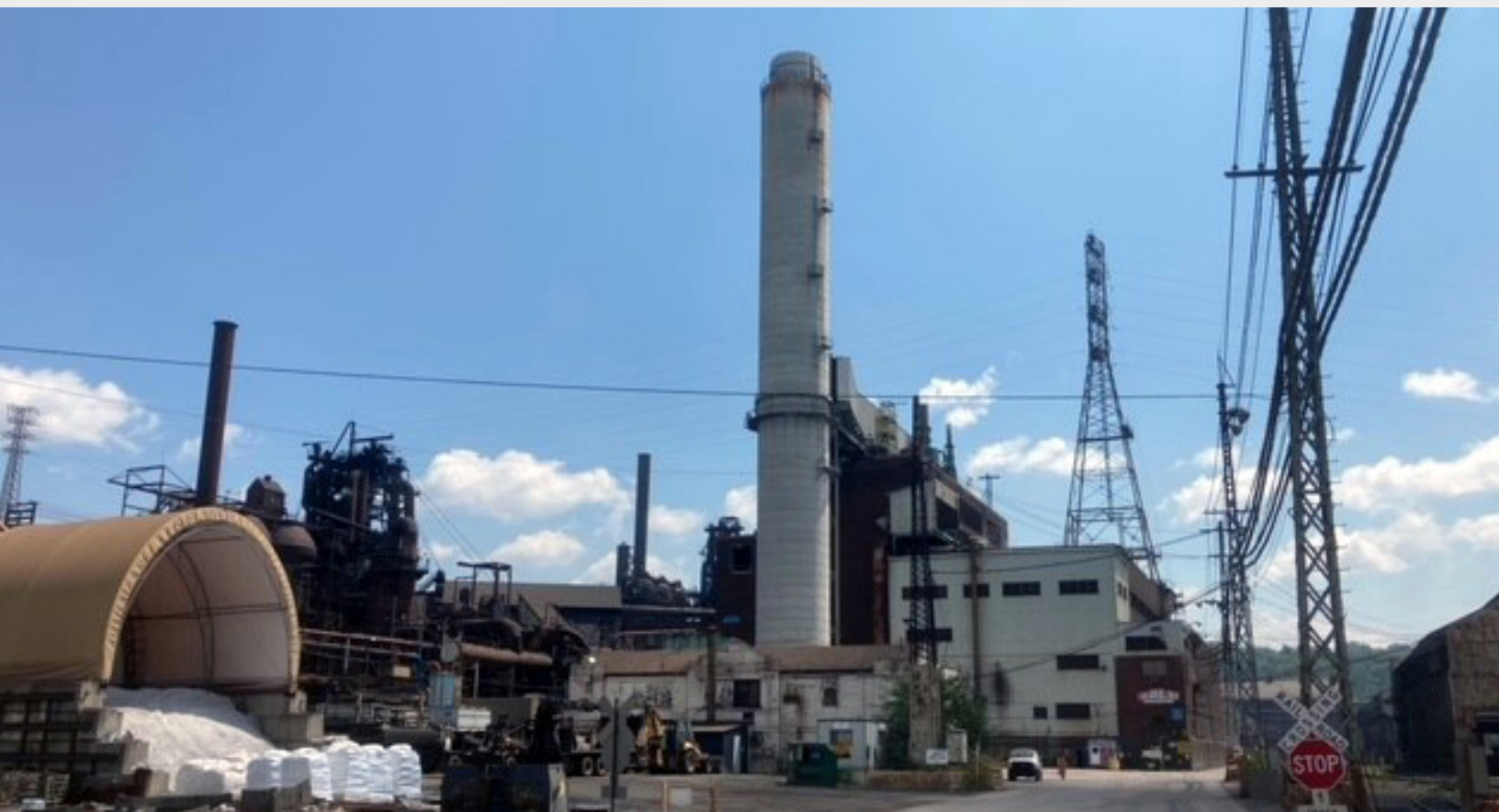
Figure 16. The Edgar Thomson Plant boilers.
