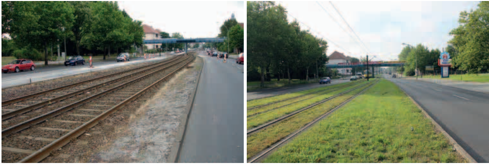
Figure 4: Appearance of the tracks before and after the greening process in Berlin (Pictures: [3]; [32])
