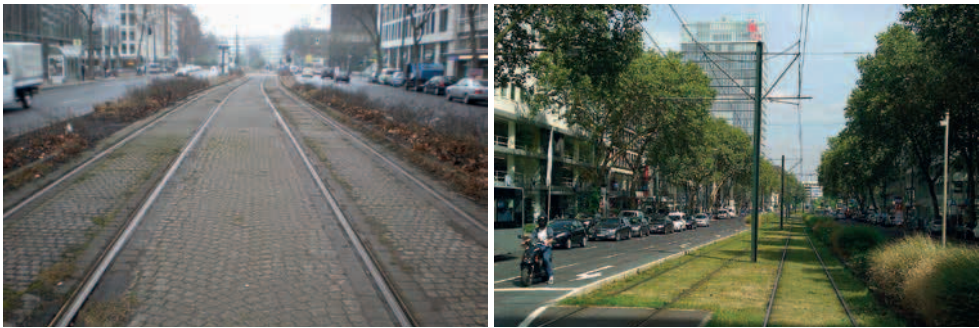
Figure 5: Appearance of the tracks before and after the greening process in Düsseldorf (Pictures: [1])
