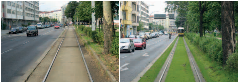
Figure 6: Appearance of the tracks before and after the greening process in Berlin (Pictures: [12])
