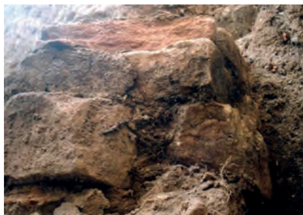
▲ Fig. 2. Stará Boleslav. Remnants of the 10th century defensive wall built of sandstone blocks bound with mortar ( opere Romano ). Photo I. Boháčová.
