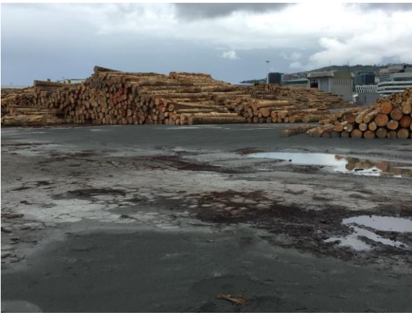
Figure 11: Sandy liquefaction ejecta in the log stacking area (hydraulic fill reclamation) in the northeast corner of CentrePort (Sample S13). (S41.274972° E174.788347°, taken on 17 NOV16).
