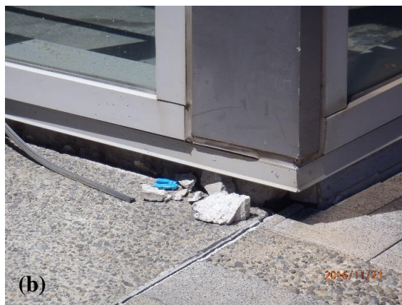
Figure 36: Ground settlement relative to the pile-supported B building at: (a) the southwest corner of the building with ground improvement (S41.279767° E174.782100°, 21NOV16), and (b) northwest corner of the building without ground improvement (S41.279419° E174.781443°, 21NOV16).
