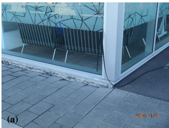
Figure 36: Ground settlement relative to the pile-supported B building at: (a) the southwest corner of the building with ground improvement (S41.279767° E174.782100°, 21NOV16), and (b) northwest corner of the building without ground improvement (S41.279419° E174.781443°, 21NOV16).
