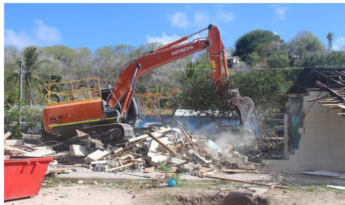
Demolition of the fire ravaged public health building on 5 January
