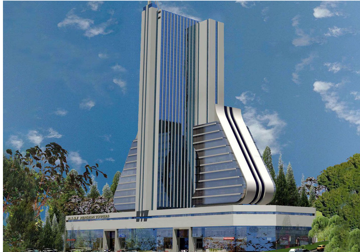
Pension Towers, commercial real estate project by the National Social Security Fund
