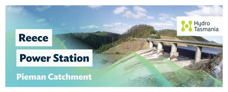
Reece Power Station is located at the foot of the Lower Pieman Dam, and is the lowest of the four power stations in the Pieman River Scheme. It was commissioned in 1987 and houses two machines comprising Francis turbines coupled to Fuji generators.
