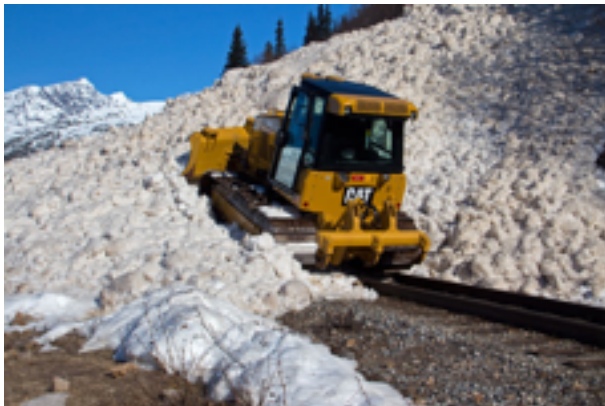
A bulldozer begins clearing fresh avalanche debris from the 15.2 Mile Path in May 2015.
