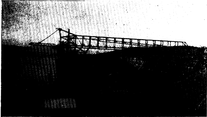
Loading dock for sinter and ore at Michipicoten Harbour.
