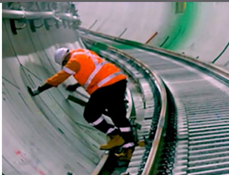
Track jacks used to lift rail to rough line and level
