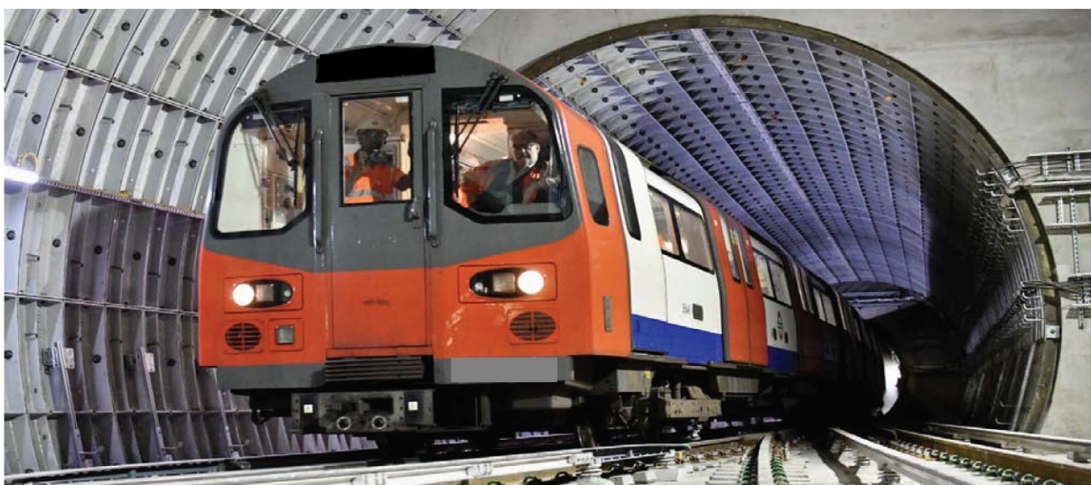
Figure 4: London Underground Kennington Loop SGI step plate junction
