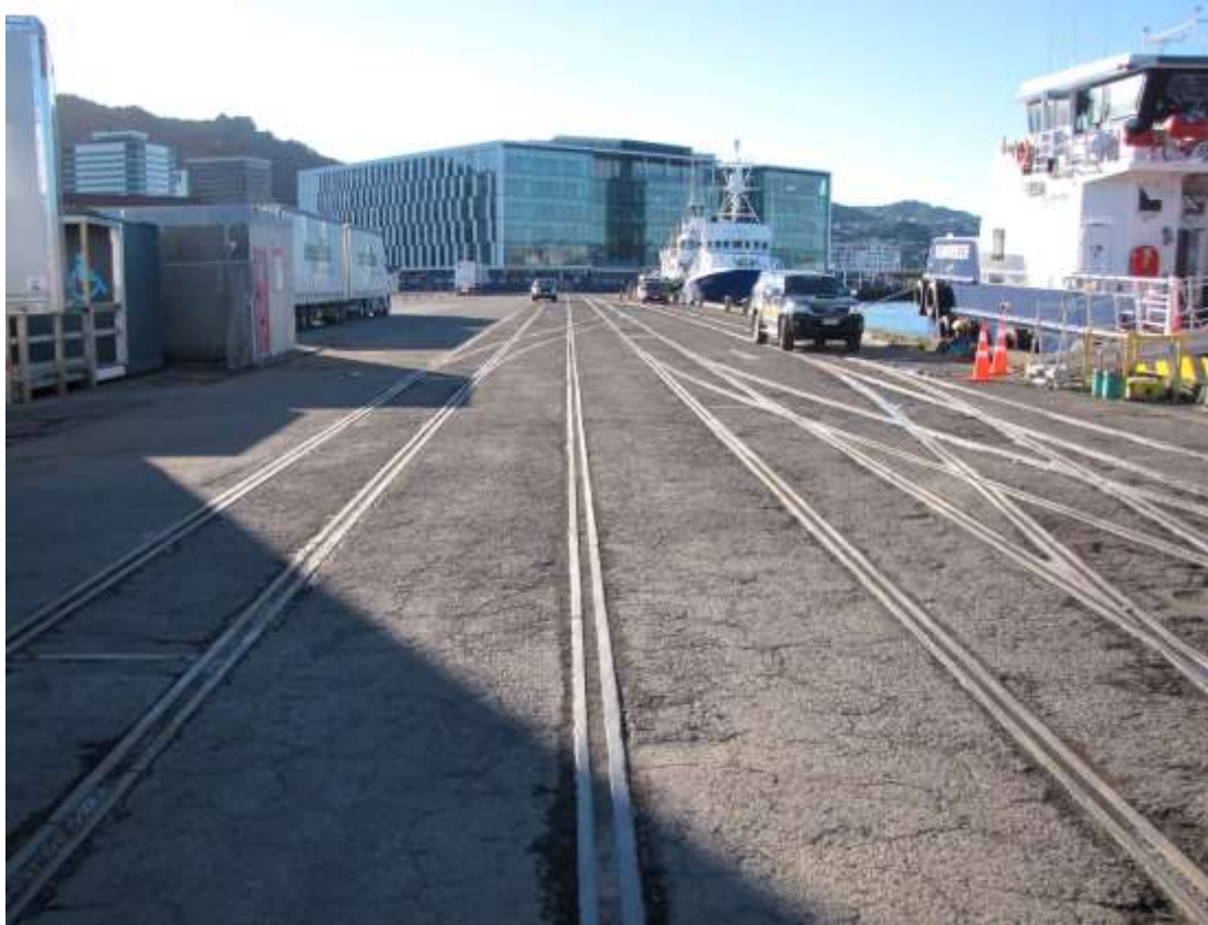
The deck of Glasgow Wharf, looking north to the landward end.
