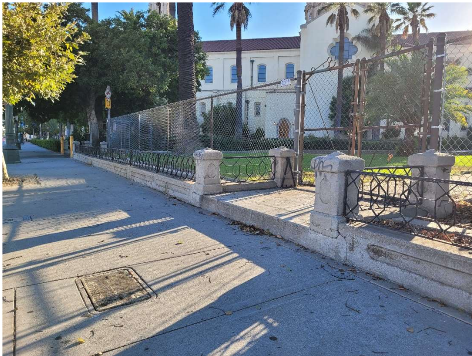
Figure 10. Pedestrian bridge and Zanja No. 8-R, view south.
