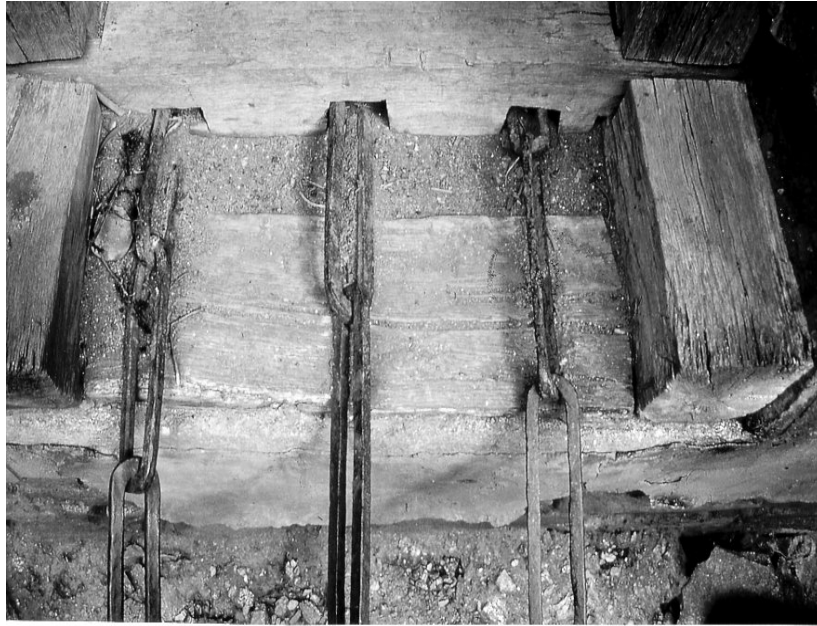
Fig. 35: The anchorage of the Doksum Chakzam
