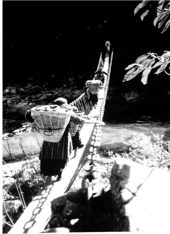
Fig. 40: Iron chain bridge across the Bhoté-Kosi in Nepal. Photo: Hans Renatus
