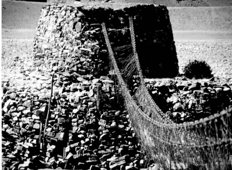
Fig. 26: The part of the Phuntsoling Chakzam across the Yarlung Tsangpo, which is still functioning.
