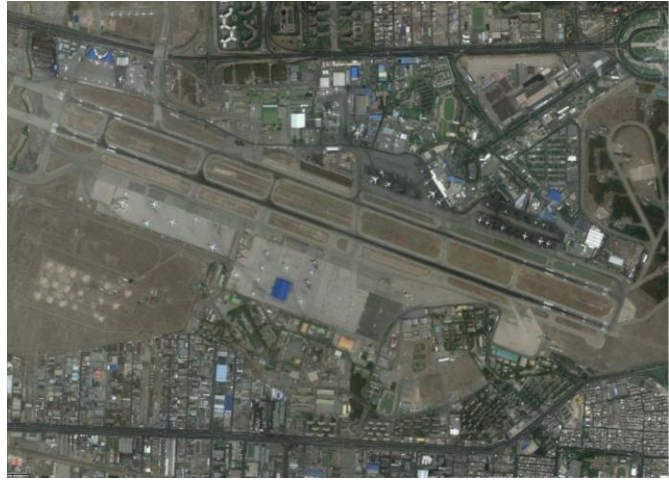
Tehran Mehrabad Airport, Tehran Iran, GoogleMaps, 2009
