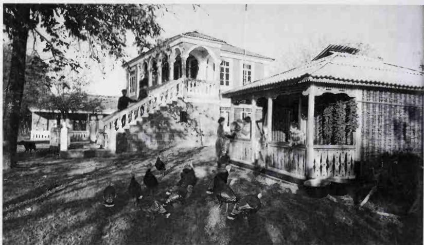
Popular arrangement of buildings in a village homestead: main dwelling, often with external stairs, outhouse and replica of the ancient wattle structure (a'patsxa) in the foreground
