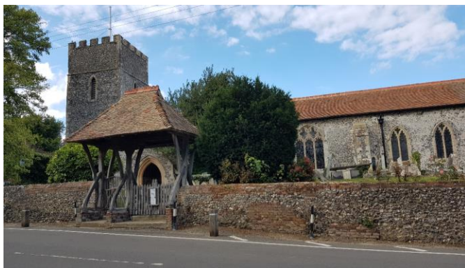
Church of St James, Staple (Grade I listed)
