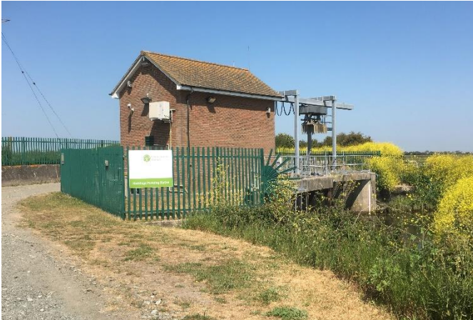
Hacklinge pumping station
