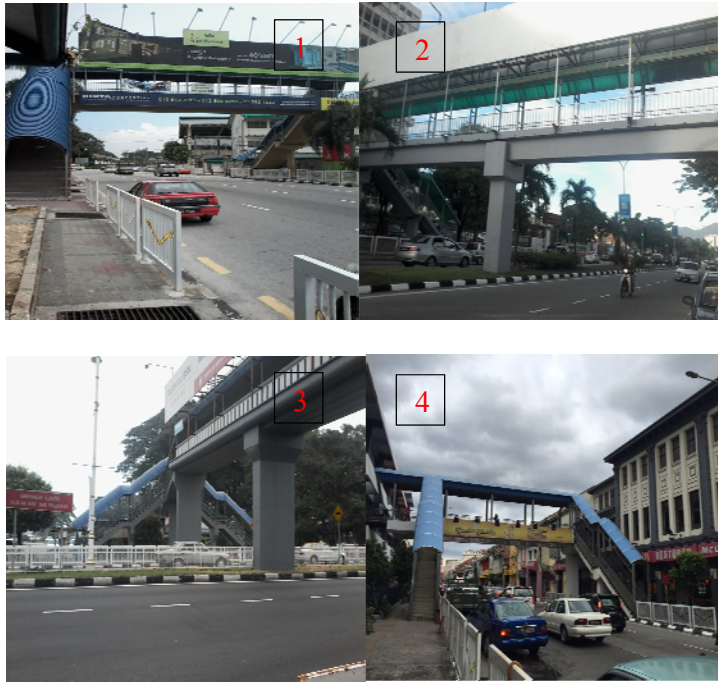
Figure.1. Photos of the footbridges in Ipoh city
