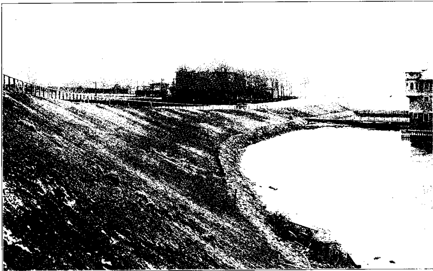
TEMPORARY WIDENING, SHORE ROAD.
