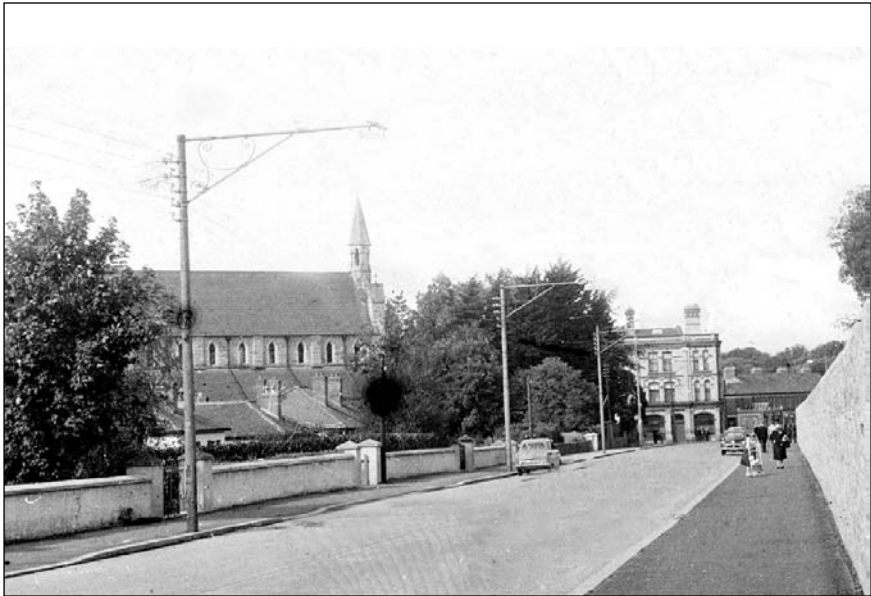
Church of the Annunciation and the Yellow House, Rathfarnham in the early 1960s.
