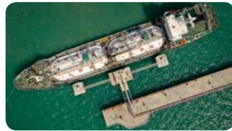
Uji coba Terminal LPG Rembang. Commissioning LPG Terminal Rembang.
