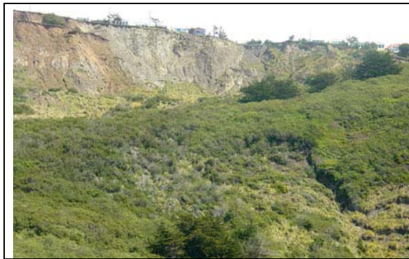
Figure 8-11. A massive landslide complex at Mussel Rock Park masks the main trace of the San Andreas Fault. Note the high, barren slump escarpment in the background. Ongoing coastal erosion at the toe of this slide area promotes the landward migration of the high wall of the landslide escarpment. Numerous homes have been destroyed, damaged, or condemned along this coastal slide area of Daly City.
