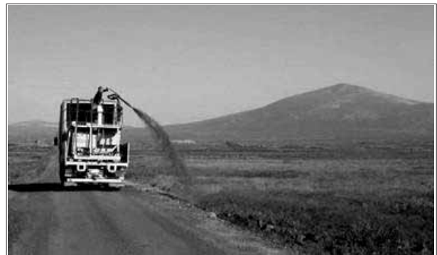
Figure 2. Hydroseeding application of commercial seed mixture at an alpine site in Norway.
