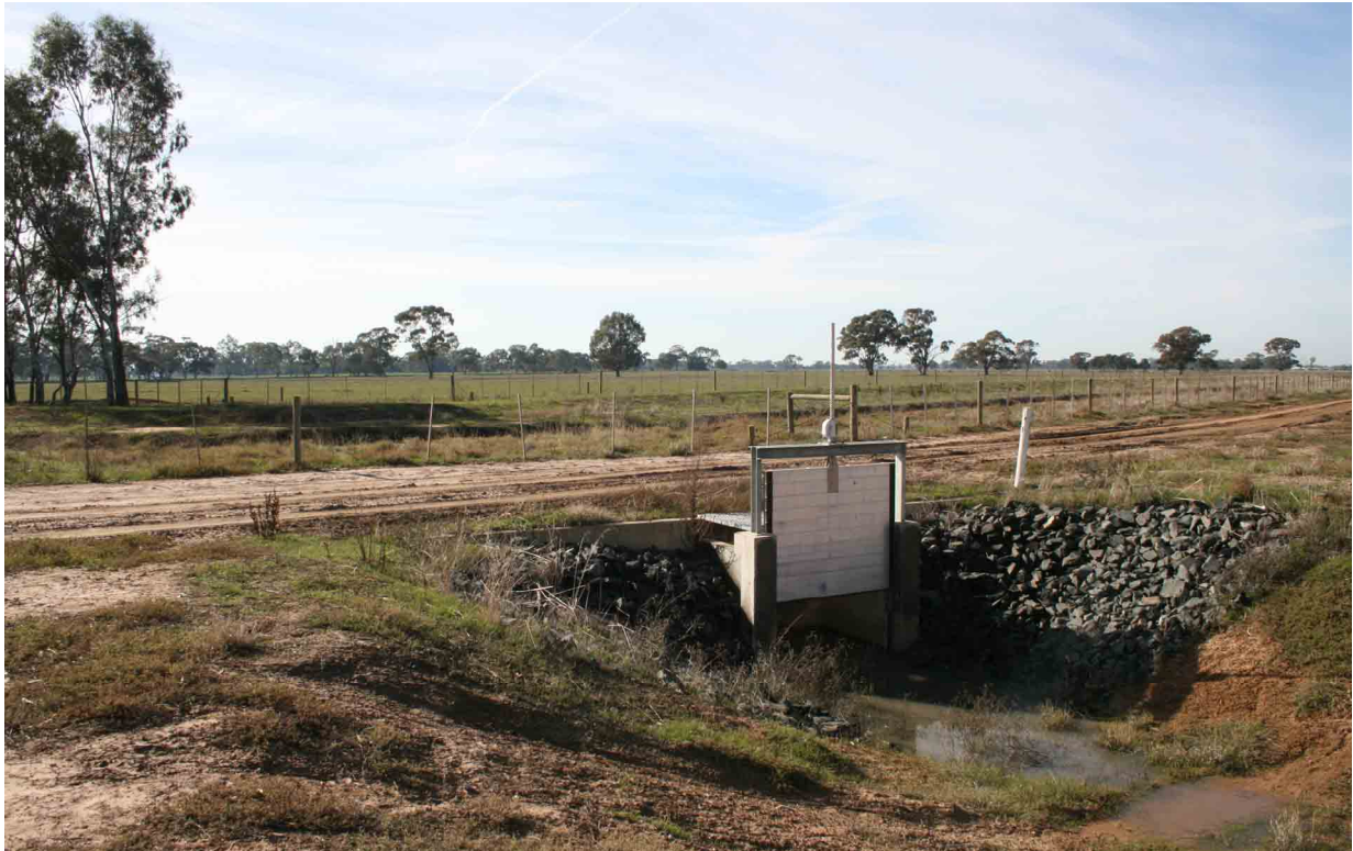
Image 8. Water regulator at Mansfield Swamp SGR in central Victoria.
