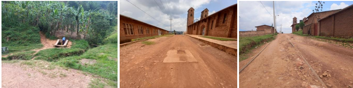
Photo 2: Water utilities in the right of way to be affected and lost
