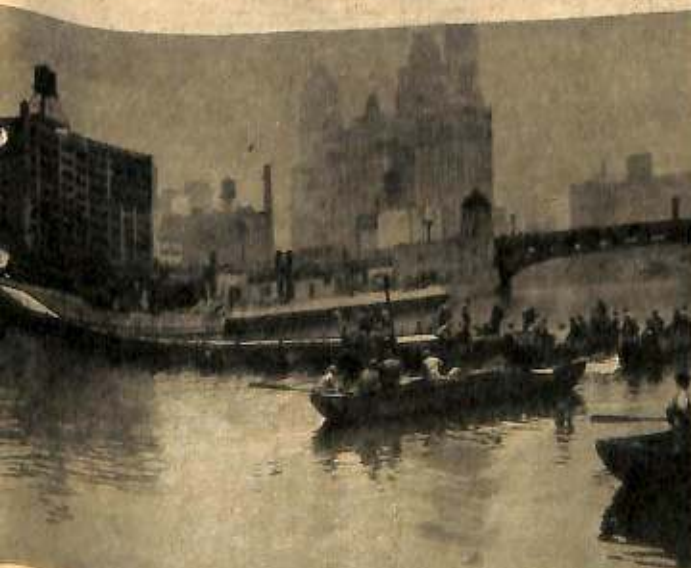
U. S. Army Engineers from Camp McCoy, Wis., built a pontoon bridge across Chicago River in less than an hour and dismantled it in another hour—a demonstration celebrating the Engineers' 168th Anniversary.
