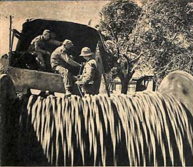
SALVAGED WIRE is being rewound on cable drums by men of Construction Battalion.
