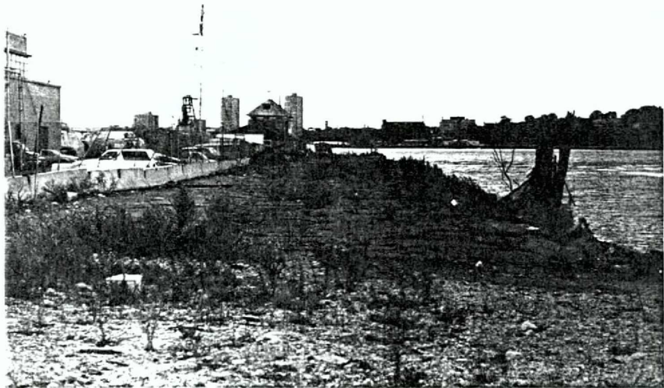
PHOTO C: Pier 53 (facing west).
