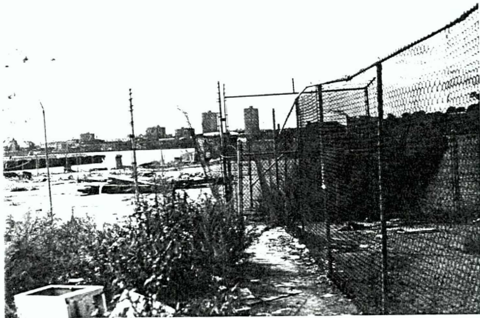
PHOTO E: Foot of Pier 57 (facing northwest).
