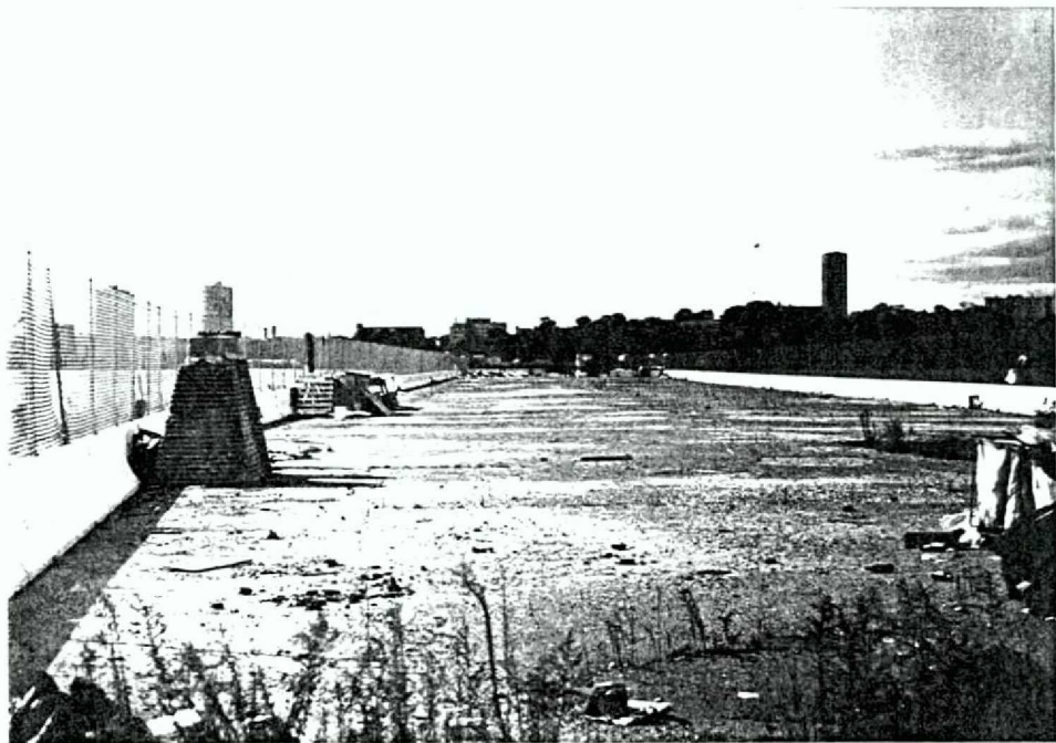
PHOTO D: Pier 56 (facing west).
