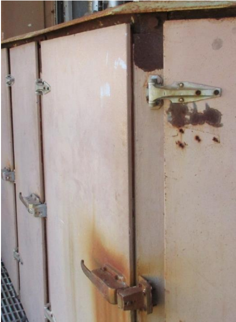
Figure 3-7 — Lack of GT Enclosure Sealing
