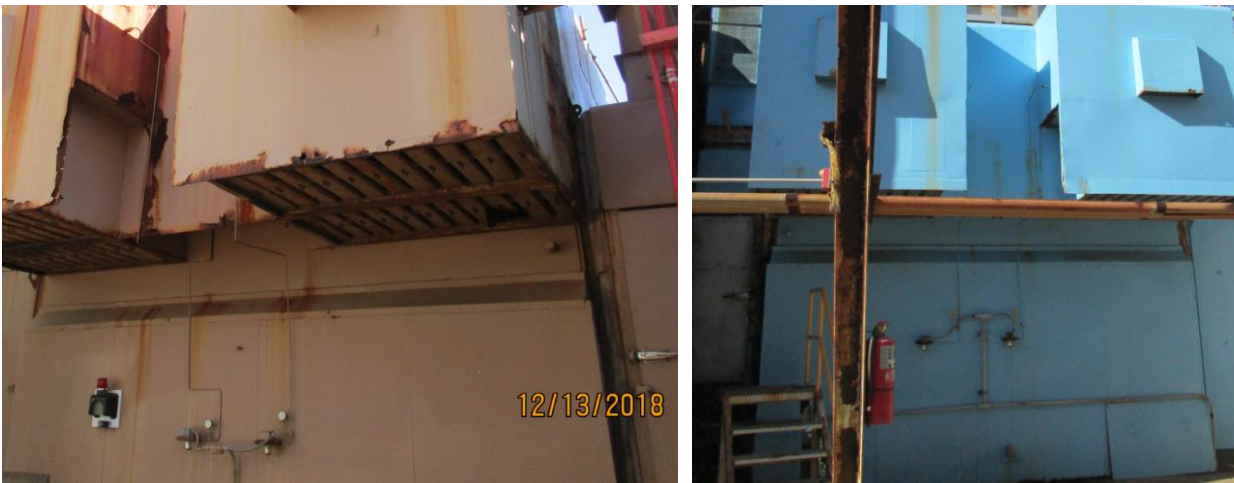
Figure 3-39 — Refurbishment of GT Generator Filter Cabinets
