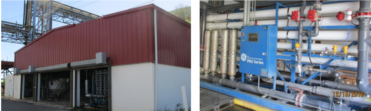
Figure 3-20 — Water Treatment Building
