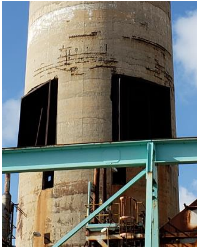
Figure 3-10 — Abandoned Concrete Stack
