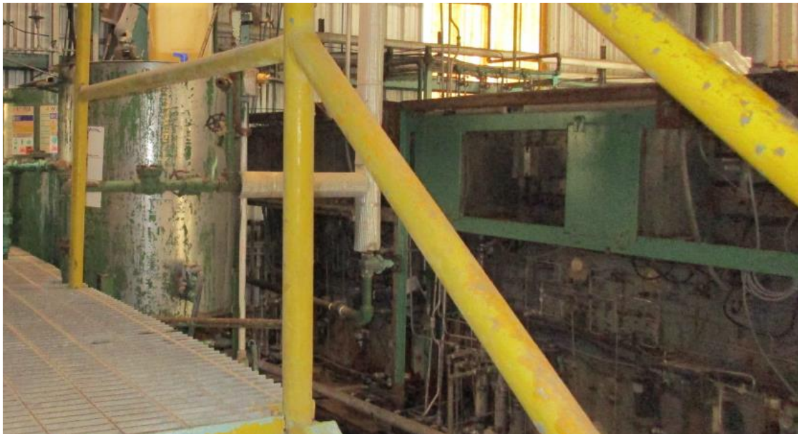
Figure 3-21 — Demineralizer at CC Unit
