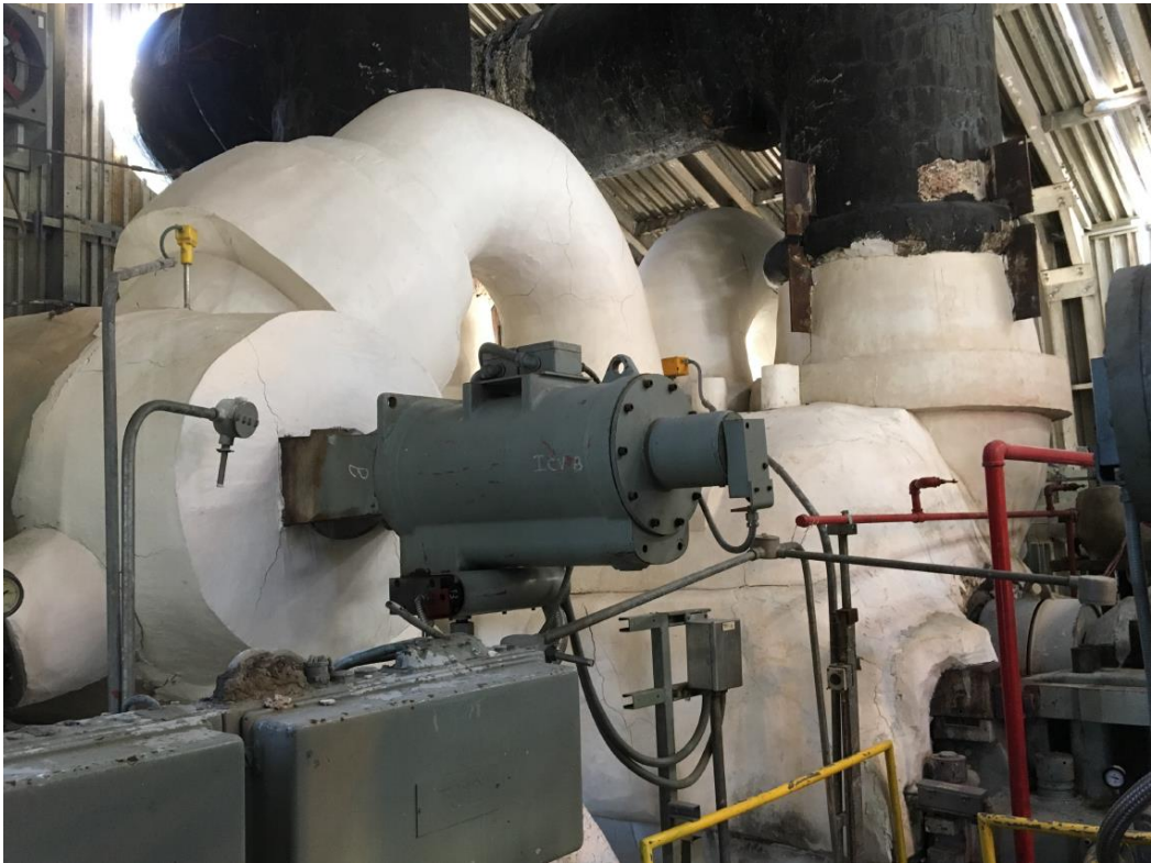
Figure 3-3 — Unit 2 STG IP Section
