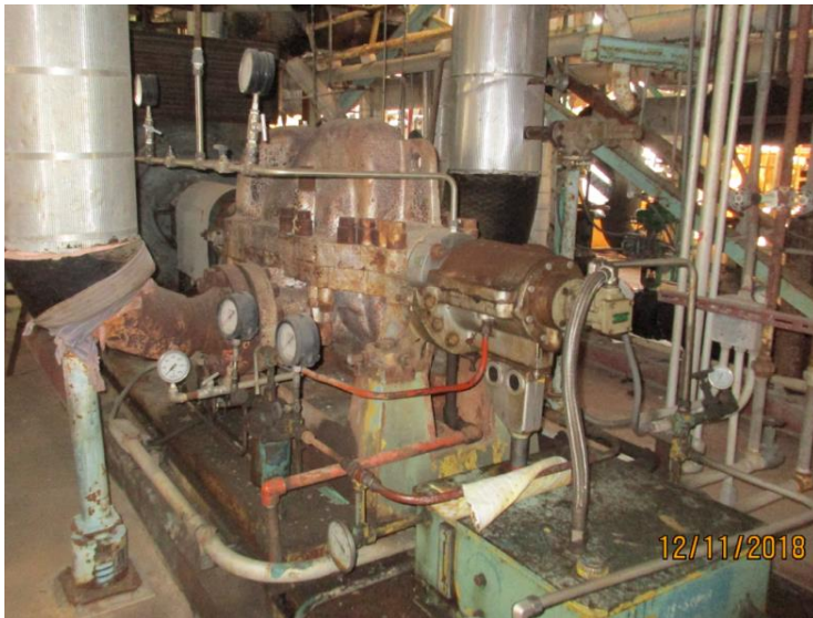
Figure 3-14 — Combined-Cycle BFPs
