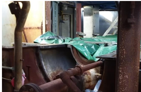
Figure 3-8 — GT 2-2 Compressor Rotor Storage and GT Housing Layup
