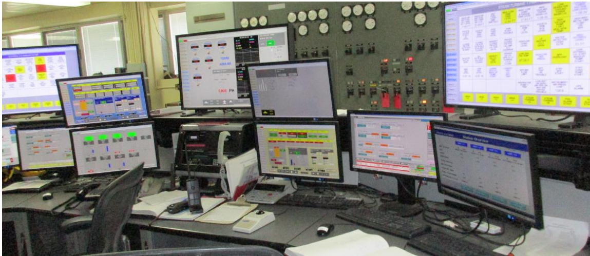
Figure 3-34 — HRSG Control Room – Foxboro Upgrade in Progress
