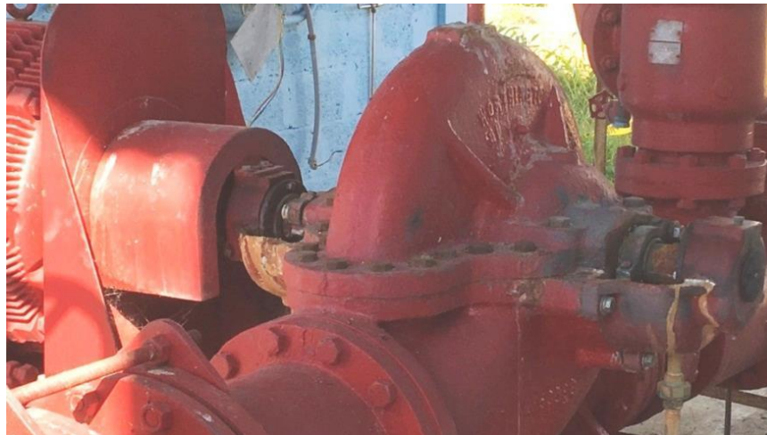
Figure 3-25 — Electrical-Fire Pump
