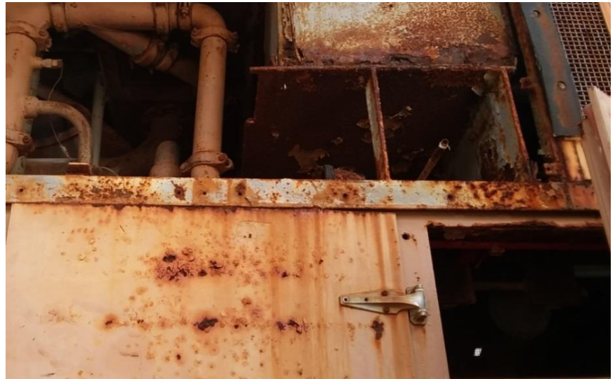
Figure 3-7 — Lack of GT Enclosure Sealing
