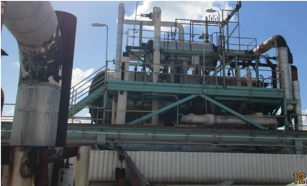
Figure 3-14 — Combined-Cycle BFPs
