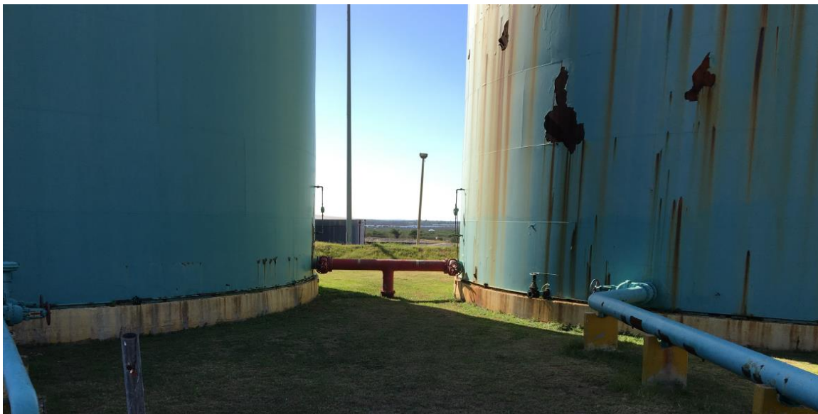
Figure 3-19 — Well Water Tanks
