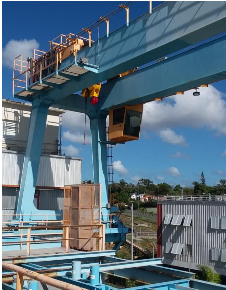
Figure 2-4 — Turbine Deck Gantry Crane, Units 1 and 2
