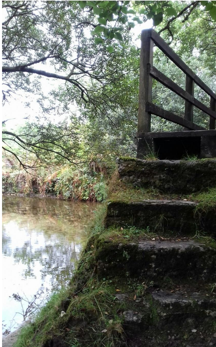
Figure 5.32 Bridge over river Fowey, Carneglos (Source: author)
