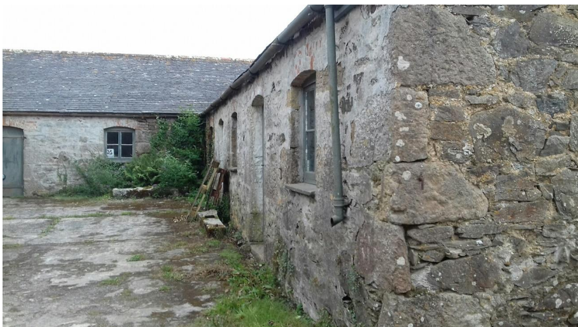
Figure 4.32 Gear Farm settlement, showing building overlying small round (Source: author)
