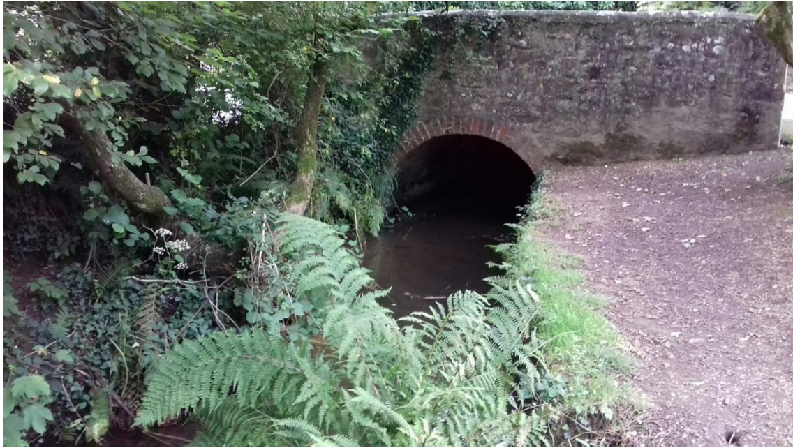
Figure 5.26 Bridge over river Amble tributary (Source: author)
