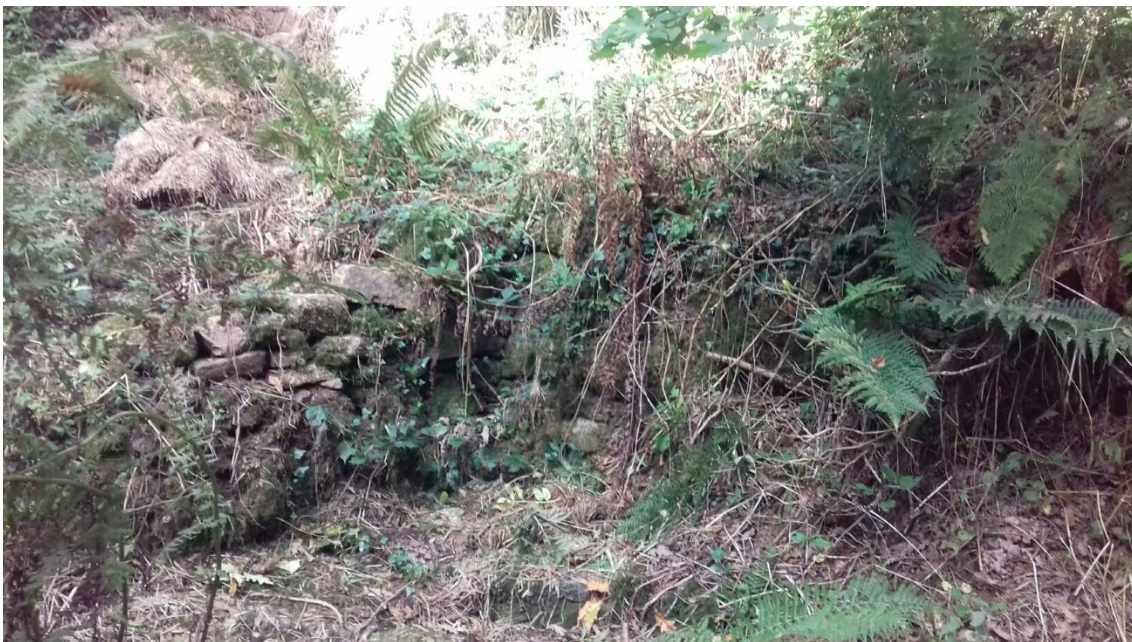
Figure 6.18 Fenton-la chapel walls, looking northeast (Source: author)
