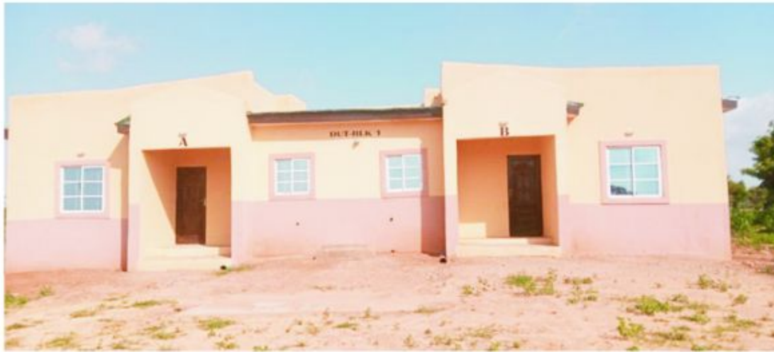
sample of 4 Constructed Low Cost Housing Units of 2-Bedrooms across the State
