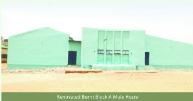
Renovated Burnt Block A Male Hostel
