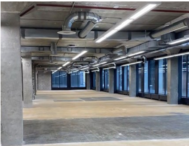
300 Sparks Street 2nd Floor in Base Building Condition
