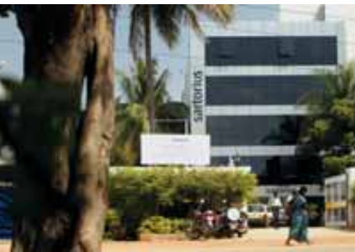
In Bangalore, India, bioreactors, fermenters and filter systems are manufactured for the Asian market.
