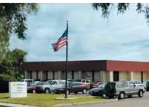
In Arvada, Colorado, USA, balances, scales, moisture analyzers, pH meters and calibration weights are produced.
