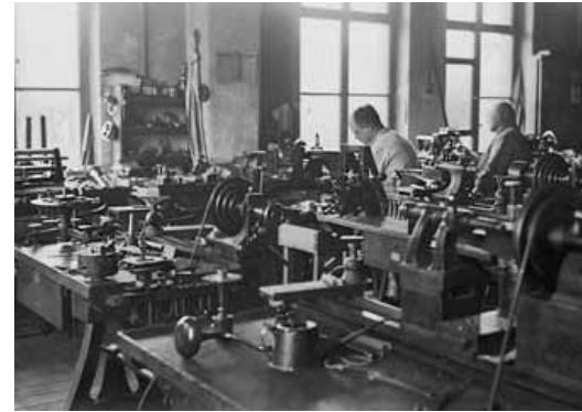
Department for microtome assembly at the second factory in Rauschenwasser, Göttingen
