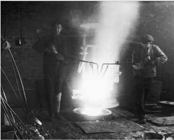
Crucible furnace in the foundry
