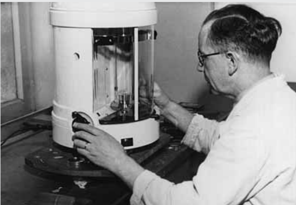
An employee calibrating and adjusting a SELECTA series balance
