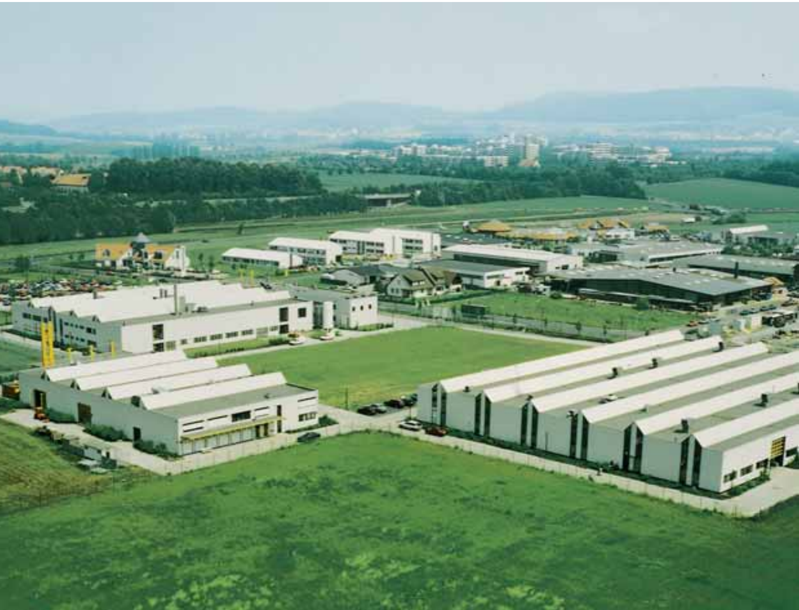
The "New Plant" ("Werk 2000"); first construction stage, 1990
