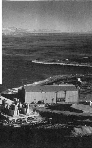
Figure 12 Portable atomic power plant, PM-3A. Above, section of plant being unloaded at McMurdo Sound in Antarctica. Below, general view of completed installation.
