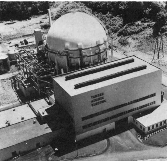
Figure 11 The Yankee Atomic Electric Station, a 175,000 kilowatt installation near Rowe, Massachusetts, was the first electric generating plant to be built under the Atomic Energy Commission's Power Demonstration Reactor Program.
