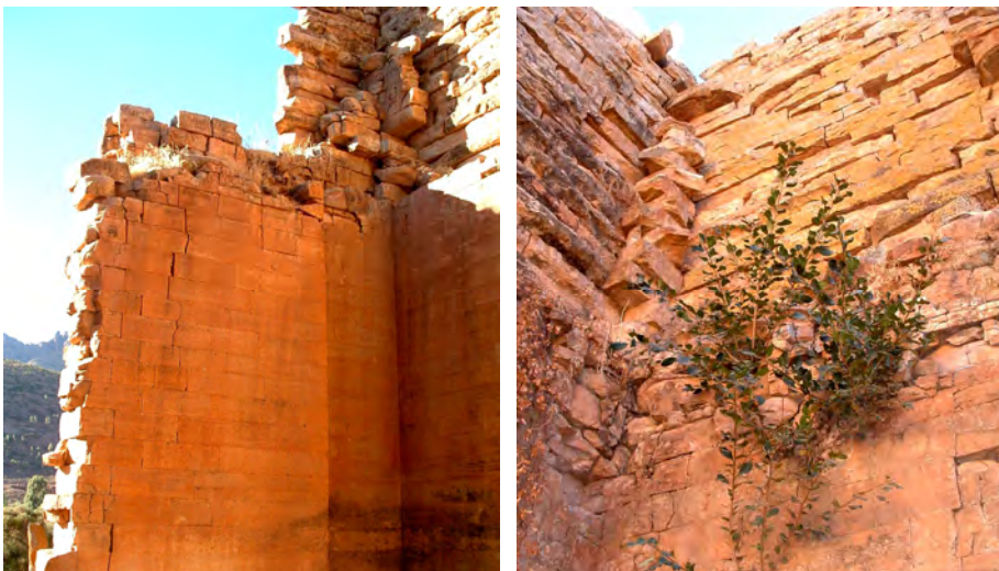
Figure 5. View of the interior walls of the Temple indicating that they were built of another layer of equally well-dressed blocks as those of the exterior wall.
