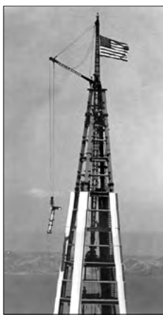
Boswell looks down after installing a Christmas tree and the American flag to the last steel beam atop the Transamerica Pyramid in San Francisco. March, 1972. Below: Photo courtesy Kaiser Permmanente.org.
